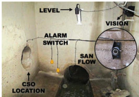
Camera, Flow, Level and Alarm Sensors are all connected to one wireless monitor running off the same battery and wireless data logger.
